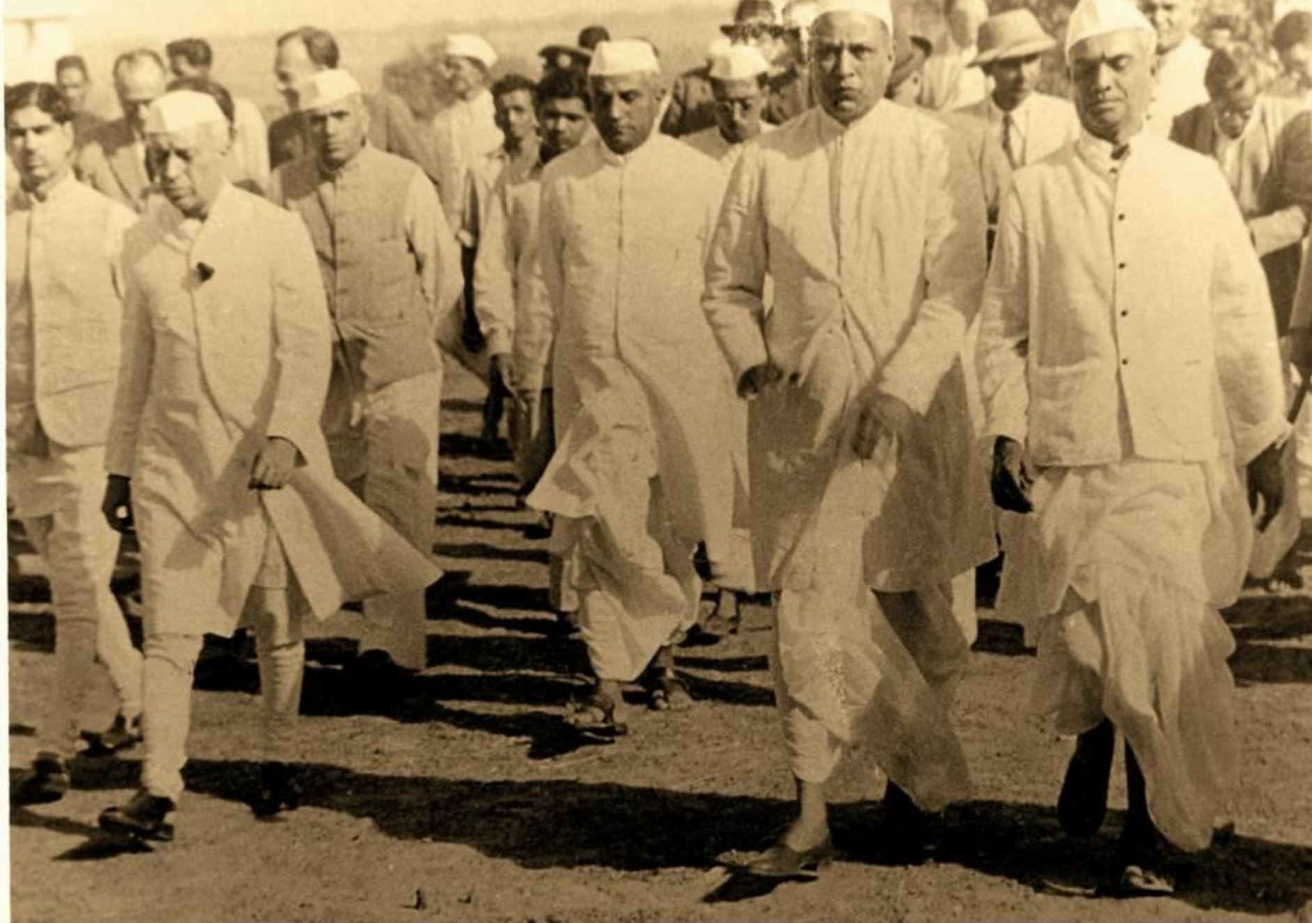
A moment of historic significance
